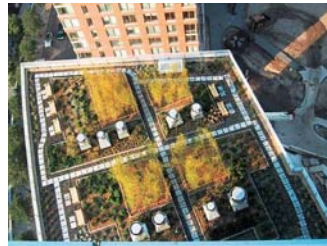
The Solaire, NYC (Image: Metropolis Magazine)
