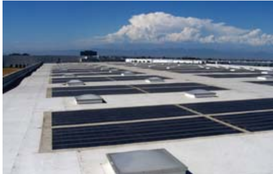
Roofing and installation of daylighting systems
