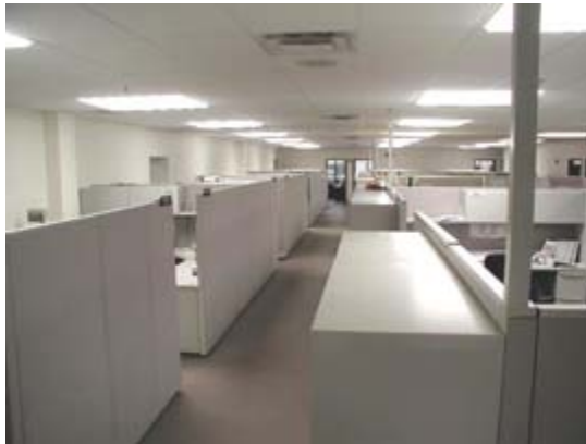
Passive daylighting and T-5 4-lamp hybrid system with integrated lighting controls daylighting only.
